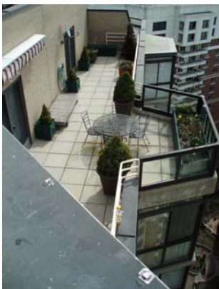
Photo 47. Balcony and Railing
