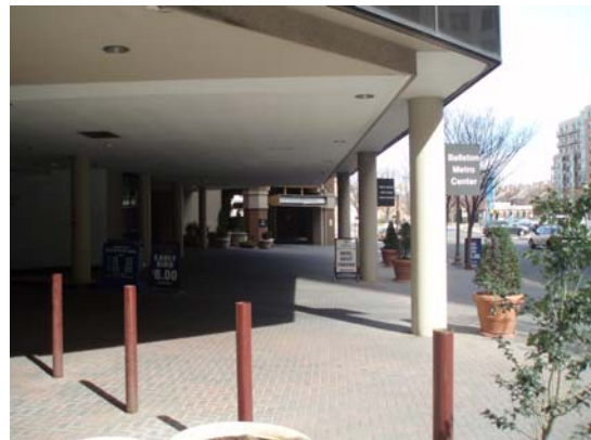
Photo 4. Walkway and Bollards
