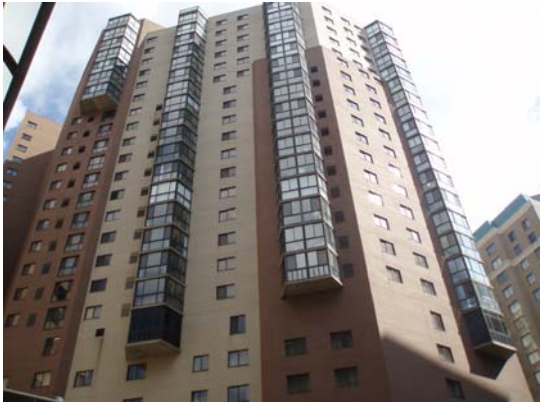
Photo 49. Bay Windows and Windows
